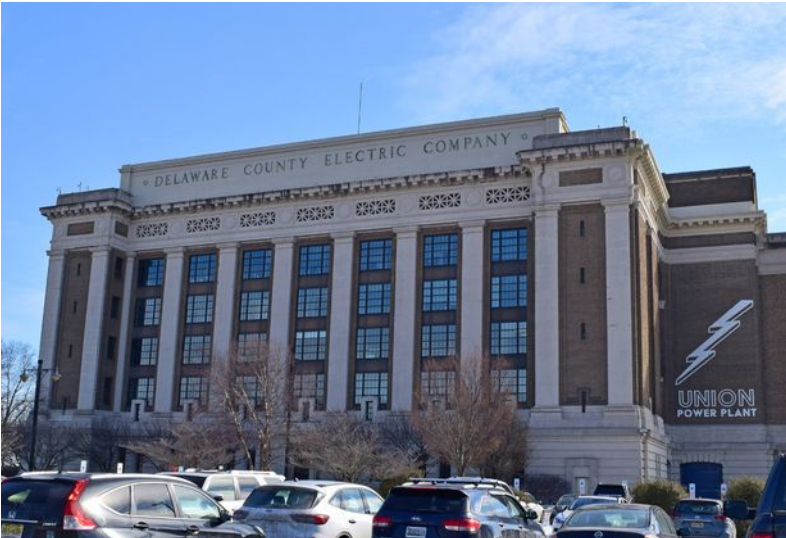
Fig. 92: Existing Chester waterfront office complex
