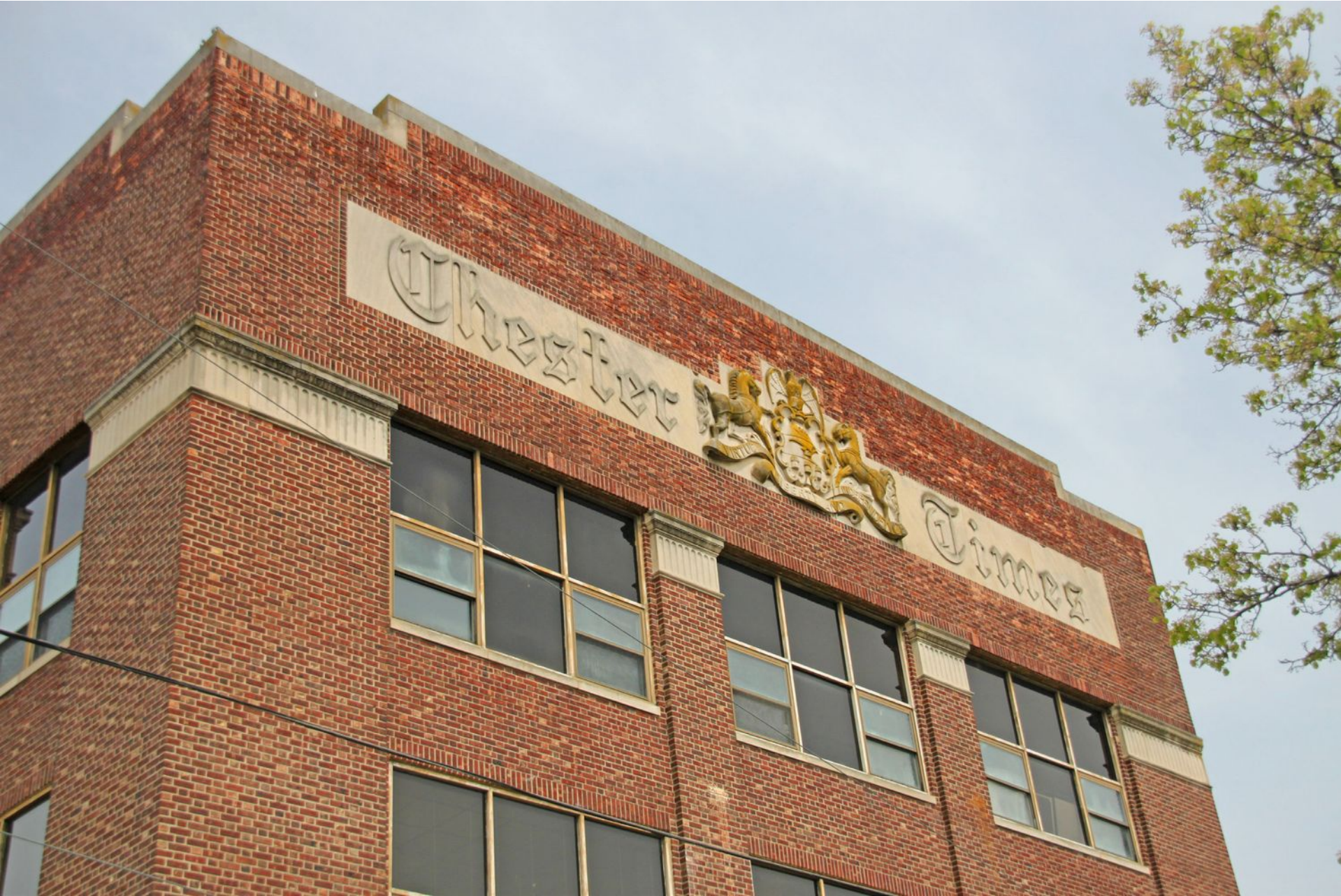
Fig. 68: Former Chester Times office building
